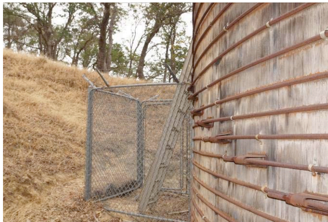
Figure 15: Tank Ladder Security Fencing
