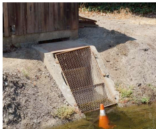
Figure 5: Pump Station Inlet Screen
